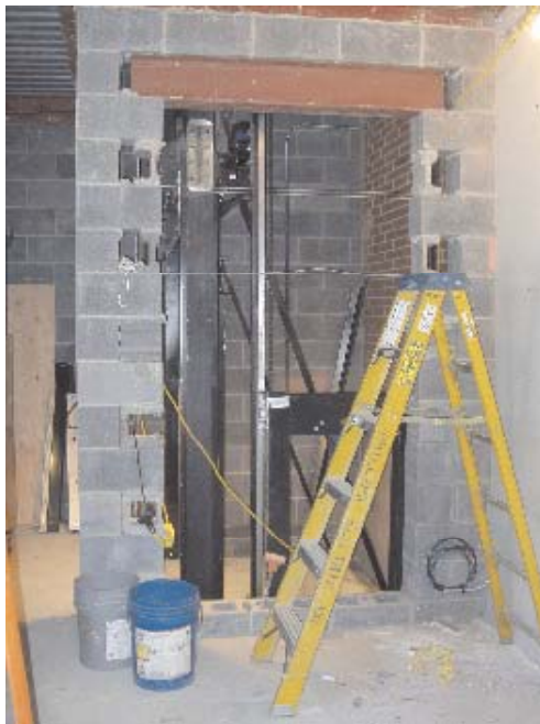
The Elevator in Progress October 6, 2004
