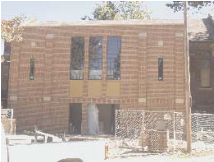
Windows and No Scaffold October 6, 2004
